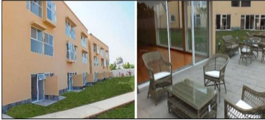
Figura 46. Espacios internos del Centro Arcadia Luxury Retirement Home
