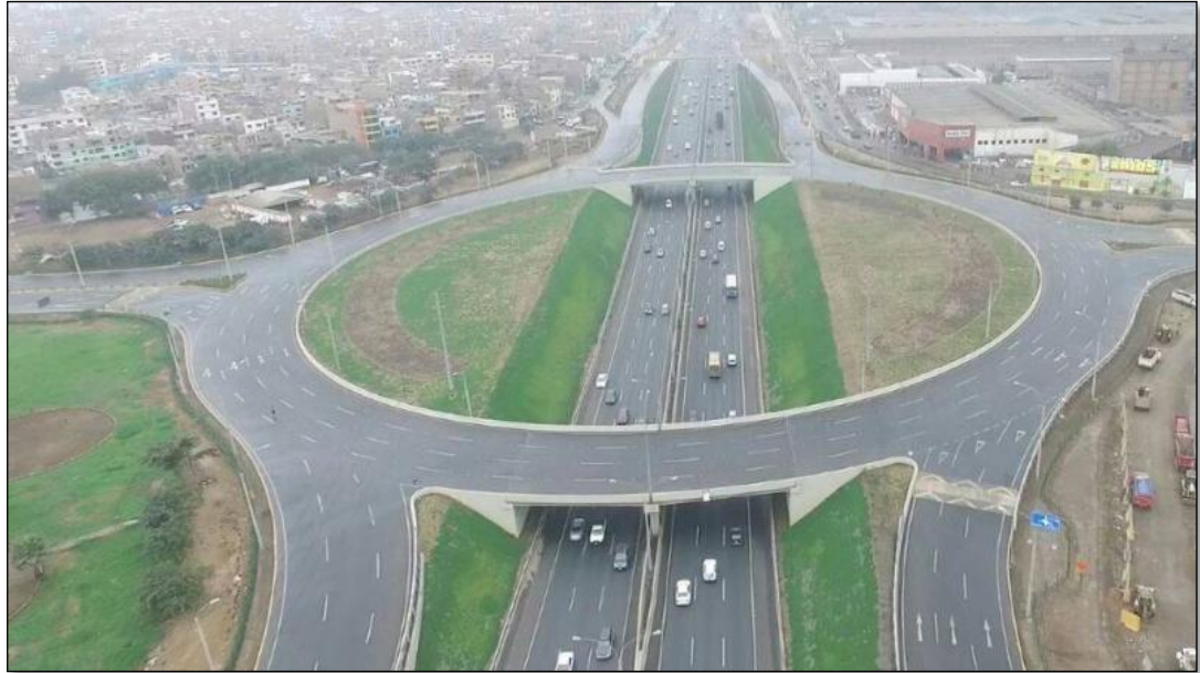
Figura 15: Intercambio Vial a desnivel Naranjal, Lima
