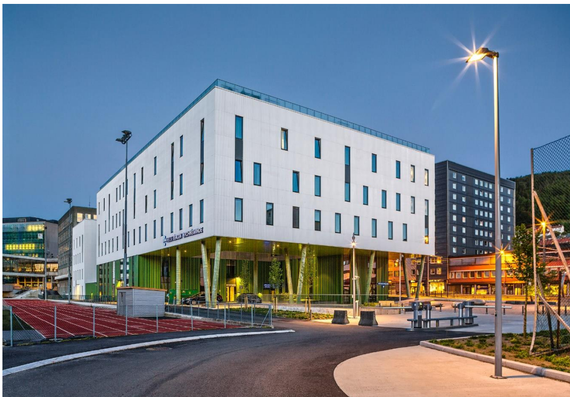
Figura N°27: Vista peatonal del Kronstad Psychiatric Hospital.
