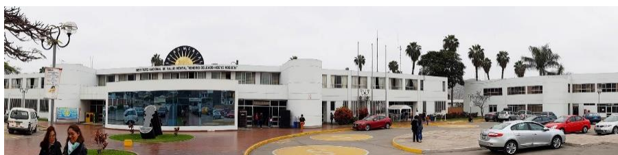
Figura N°12: Fachada principal del INHDHN
