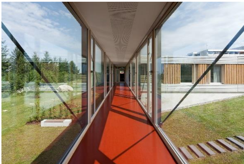
Figura N° 24, puente hospital psiquiátrico Friedrichshafe
