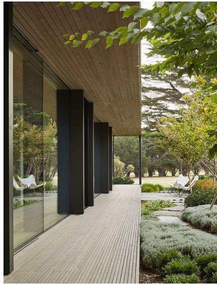
Figura 8.13: Detalle Brise-Soleil
